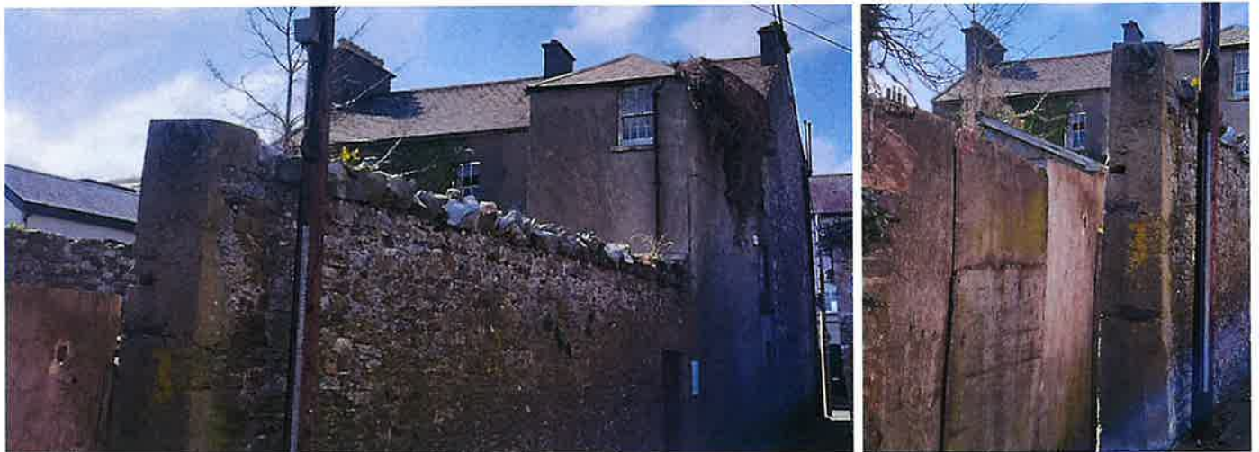
Above: Images F & G from 1 st April 2025, showing rear upper windows of 20 Church St. broken, vegetation growing from gutter and up the rear façade.
