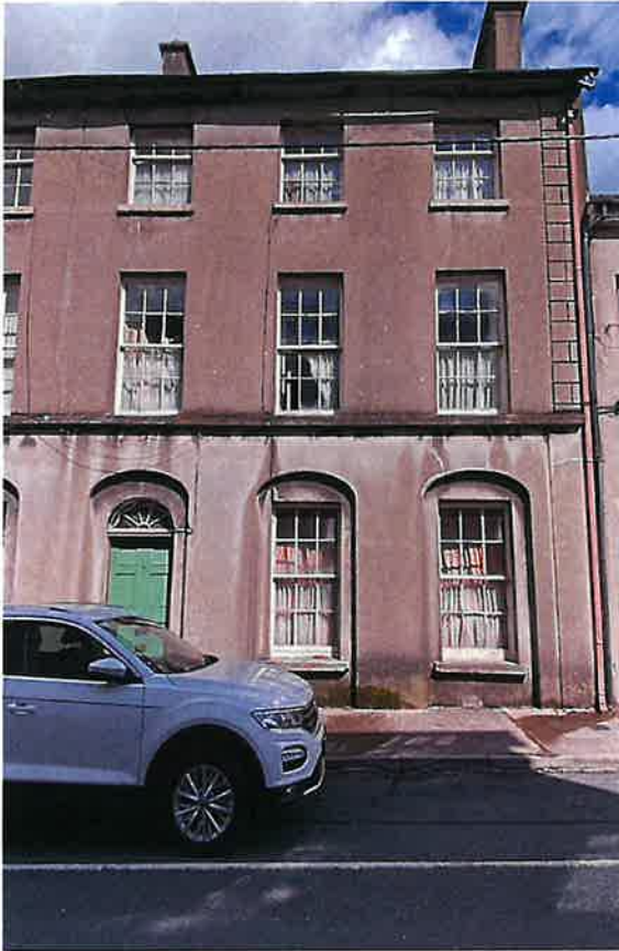
Images A & B above and images C & D below, from November 2023: Front view of the property from Church St. showing broken and damaged windows, peeling paintwork to timber windows and main doorway and poor condition and appearance of the front façade of the building.
