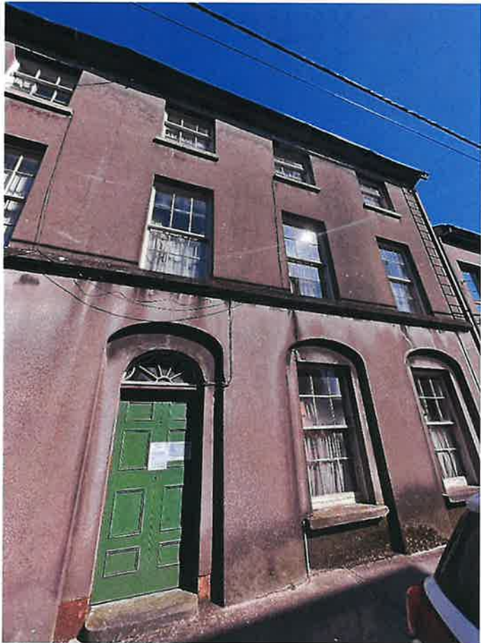
Above: Images H & I front façade showing staining and misplaced wiring & to the right, shows a window with damaged timber and paintwork.
