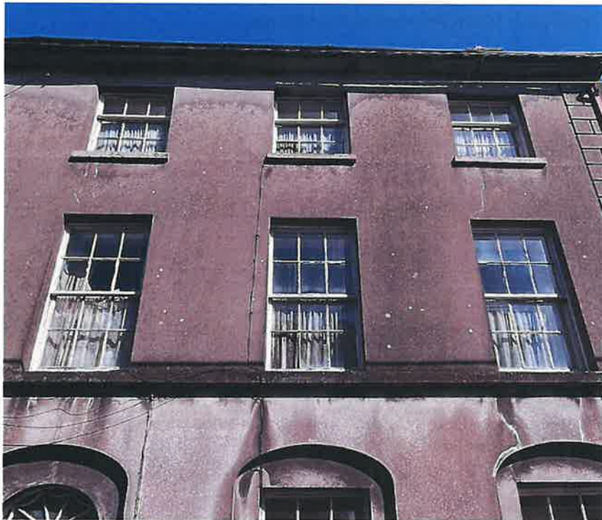
Above: Images J & K showing front façade stained and cracked, roof eaves in poor / rotting condition, first floor windows damaged / broken & showing curtains discoloured and windows in poor condition, taken from the site visit 30 th April 2025.
