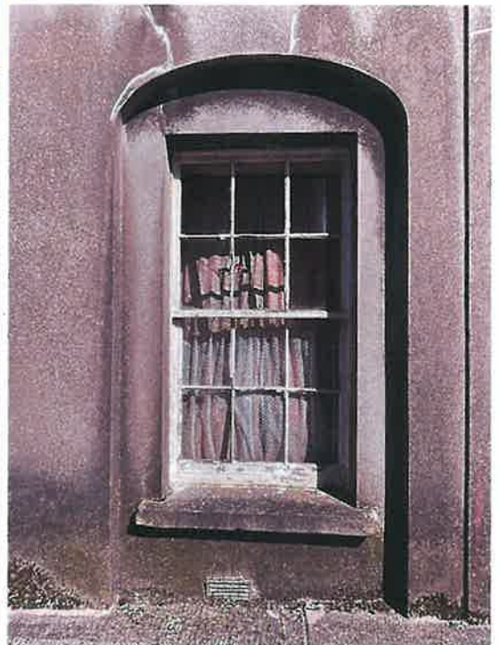
Above: Images J & K showing front façade stained and cracked, roof eaves in poor / rotting condition, first floor windows damaged / broken & showing curtains discoloured and windows in poor condition, taken from the site visit 30 th April 2025.
