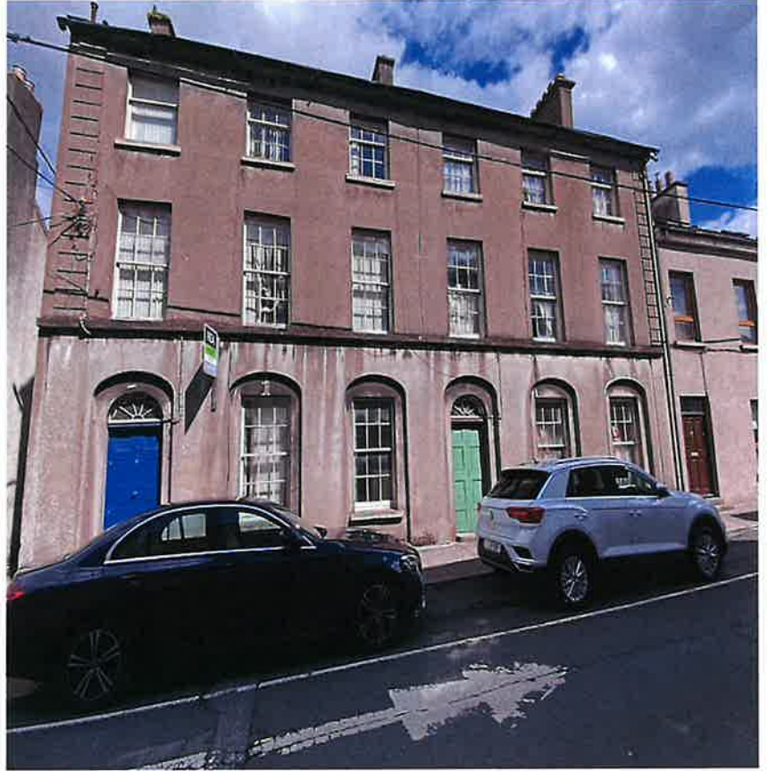
Images A & B above and images C & D below, from November 2023: Front view of the property from Church St. showing broken and damaged windows, peeling paintwork to timber windows and main doorway and poor condition and appearance of the front façade of the building.
